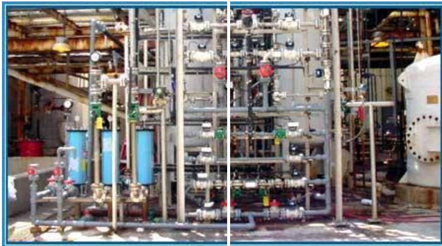
De mineralization plants are based on ion exchange technology to remove minerals from brackish water. The plant comprises of a stainless steel tank and a conductivity meter that continuously indicates the conductivity of the deionized water. Simple structure and modular design of de-mineralization plants make it easy to install. Our de-mineralization plants for use at facilities where the water contains high TDS (Total Dissolved Solid).
