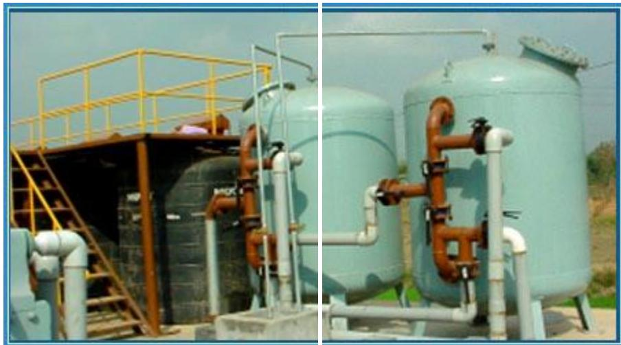
Our range of sand filters are versatile additions to industrial purification system, aquaculture, etc. These filters work by forcing water at pressure through a bed of carefully graded media that collects dirt and solids. We specialize manufacturing customized pressure sand filters in different capacities as per the client's requirement.
