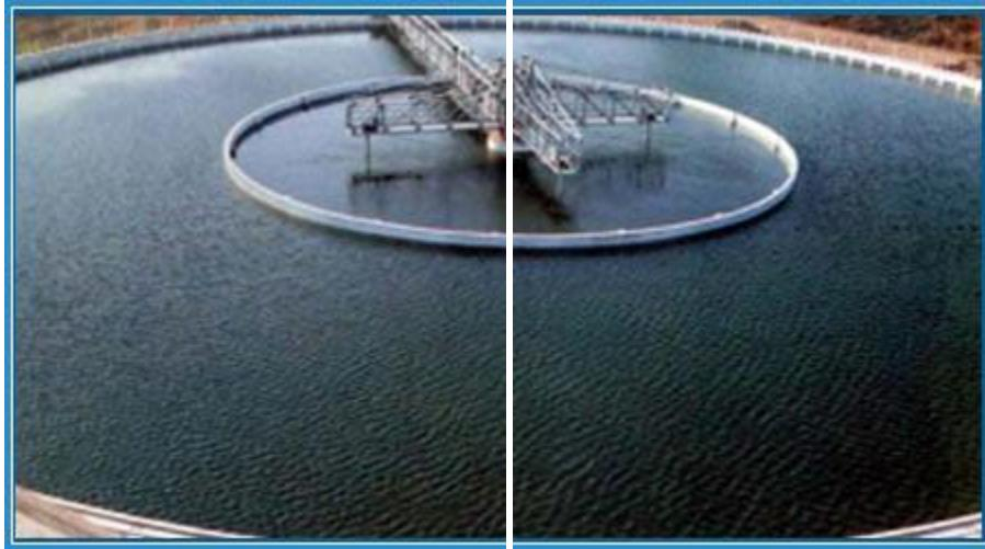
Clariflocculators are mostly used for chemical primary treatment for effluent water. These filters are designed to provide an economical and faster installation of primary treatment. The innovative design enables the clariflocculator to handle heavy slugs while delivering shortest floc settling time. Our range of Clariflocculators features high torque centre drive with sludge arm lifting device.
