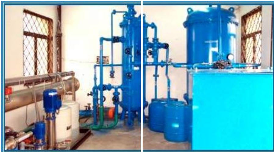
We offer highly efficient water softening plants designed to remove scale forming salts and ions such as calcium and magnesium. The softening plants are based on ion exchange process that uses resins as media. Softeners can be automatic semi automatic or largely manual as per the requirement of the clients. They are compact in size, easy to assemble, install and maintain. The unit is provided with under bed material to avoid the carryover of dirt from brine solution.
