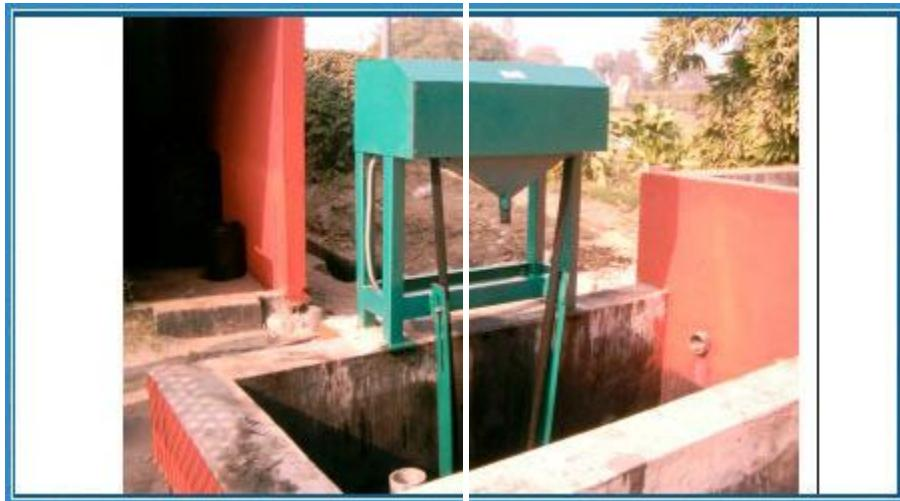
Oil skimmer or oil removal systems are widely used for removal of excess oil from sewage or industrial water. The sewage involves separation of the accumulated oil by kitchen. Kitchen absorb oil and other contaminants present in the water. In the case of industrial effluent water treatment plant, water used for washing contains oils that can be easily removed by oil skimmers. We offer different types of oil skimmers including tube type oil skimmers, belt type oil skimmers etc.
