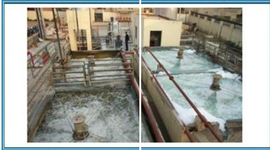
Our high quality floating aerators feature high speed rotation of the impeller to draw water. These floating aerators are equipped with heavy duty TEFC squirrel cage motors with IP-55 protection. Sturdy design enables the machine to withstand adverse weather condition, allowing for 24 hours of operation. Floats are fabricated with FRP and are filled with polyurethane foam for securing the aerators against accidental mishaps
