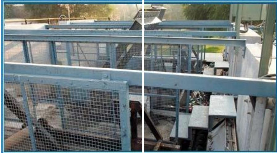
We manufacture high quality screens that are widely used for removing suspended particles from the waste water. These screens are perfectly suitable for large sewage or industrial effluent treatment plants. Screens are automatically cleaned for effective separation of suspended particle. Our engineers can also design manually cleaned coarse screens for smaller plants.
